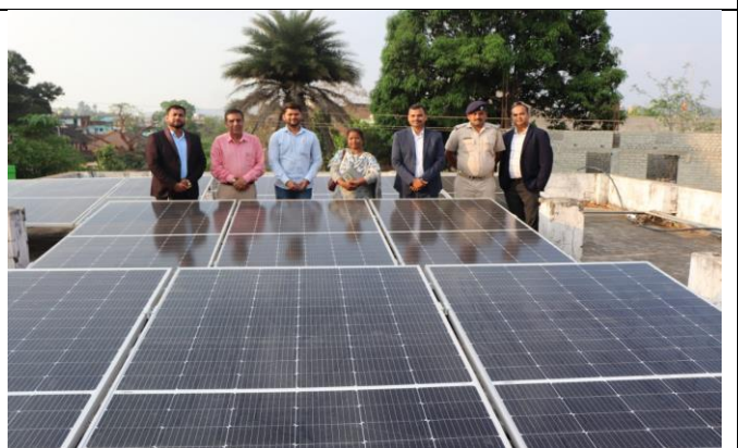
Installation of Solar Panel at Hospital at Raikia by FUSION
